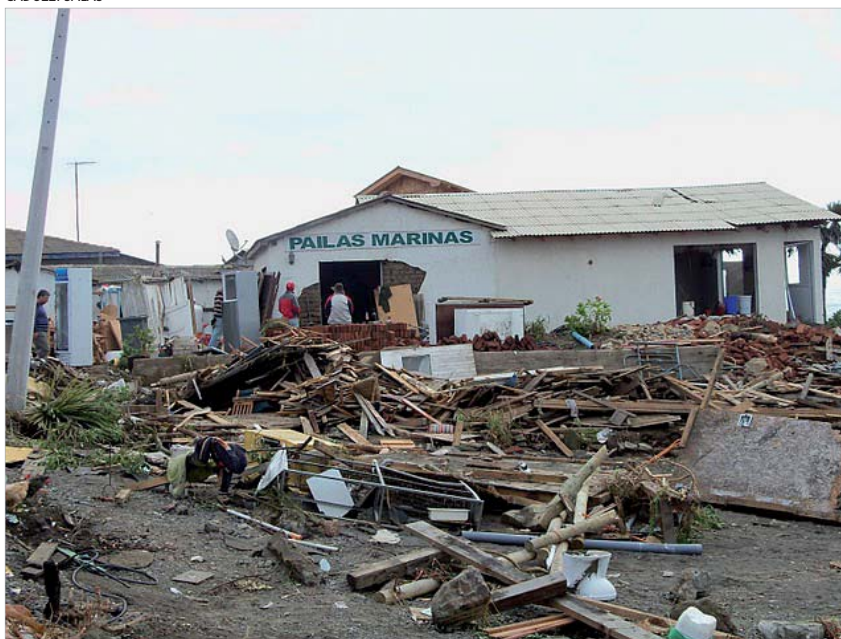
A scene of devastation from Boyeruca in the O'Higgins Region, Chile. The earthquake and tsunami mainly affected six of Chile's 15 Regions
